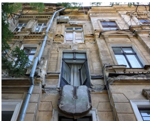
Fig. 3. Collapse of balcony slabs. Amplification schemes are wrong, correct.
